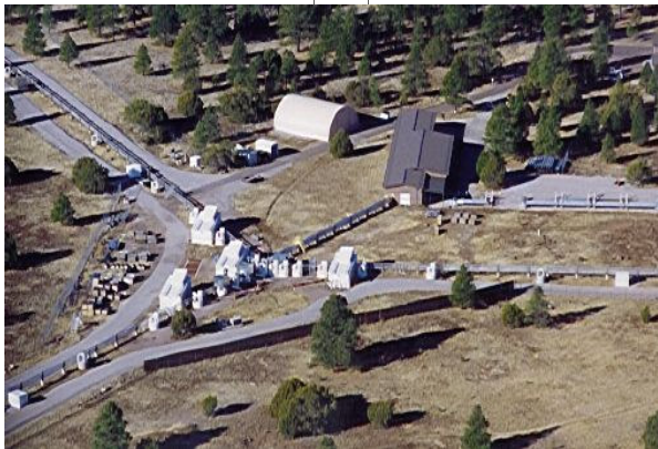
This is an aerial picture looking toward the center of the array. The four astrometric huts are visible to the left of center in the photo. The inner parts of all three arms and the perimeter road may be seen. The beam-combining laboratory is the large building visible above and to the right of center. Long-delay-line vacuum pipes are seen to the right of the laboratory.
